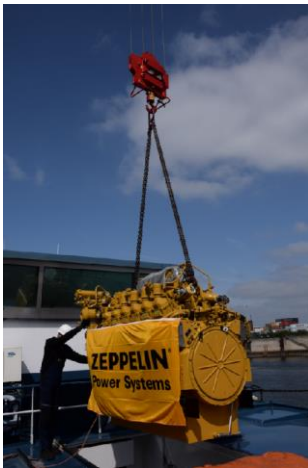
Lifting the engine down into the engine compartment is precision work.
