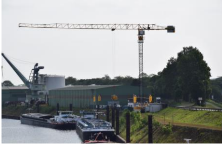
The new engine is lifted onto TMS Max using a crane.
