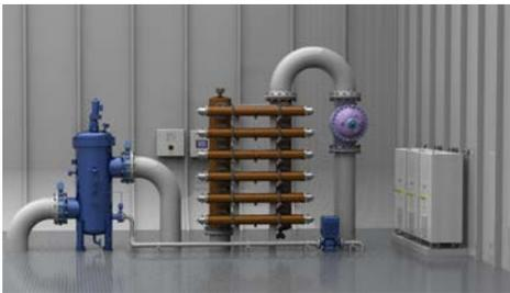
Caption: Optimarin Ballast Water System (here a 1000 m<sup>3</sup>/h solution) with systems components featuring flexible placement and easy implementation.
